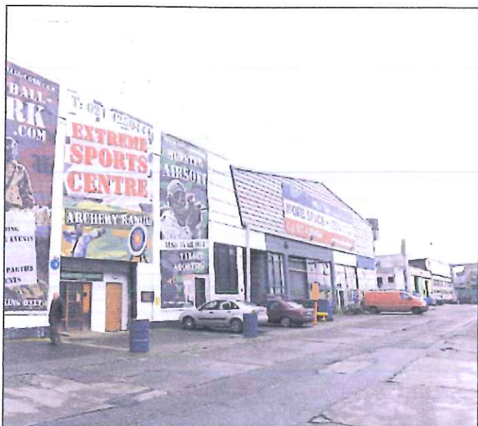
A view of Marina Commercial Park, which houses some of Cork biggest industrial lettings.
